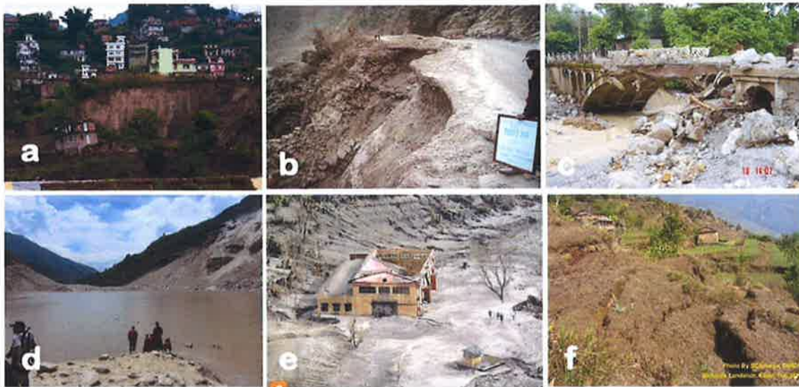
Figure 3. Landslide disaster affecting to a) Settlement: Tinthan landslide, Kathmandu, b) Highway: Mugling-Narayanghat highway, c) Bridge: Mugling-Narayanghat, d) River damming: Sunkoshi River, Jure landslide, e) Hydropower: Sanima hydropower, Jure landslide, f) Agricultural land: Sildujure landslide Kaski (source: DWIDM).
